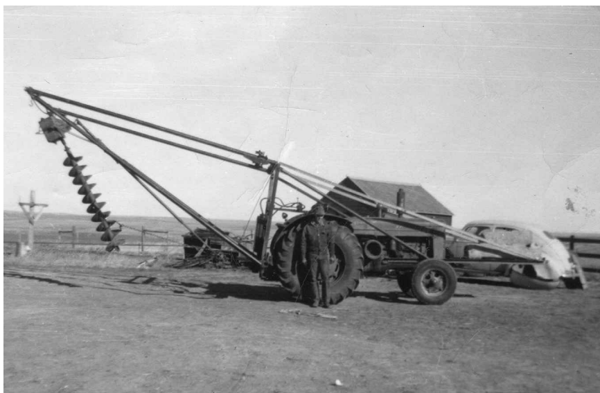
A historic photo shows a man standing in front of an auger used to dig holes for utility poles. Photo submitted by Moreau-Grand Electric
