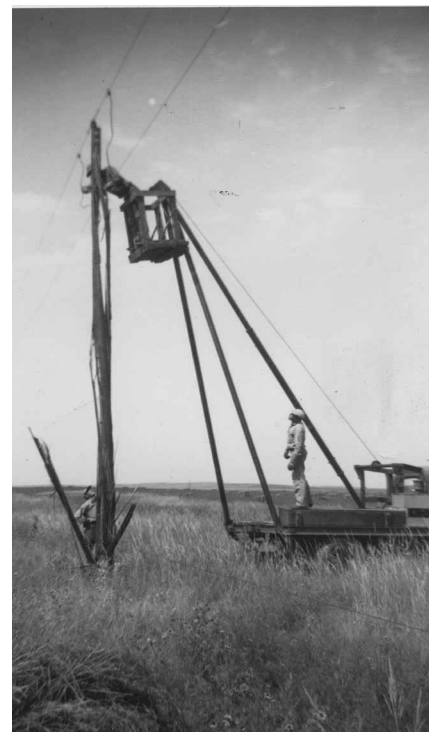
Linemen placing poles in the early days at Moreau-Grand Electric.
